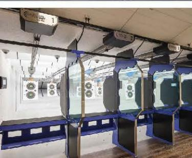
**Lighting and Electrical Installations:** Lighting and electrical installation are the most important instruments in shooting ranges, the shooting area, target and shooter sections are illuminated with different features and each section is designed to be commanded separately. In addition, the planned lighting systems are protected with angled manufactured protection steels that will not bounce or pass the bullet cores.
